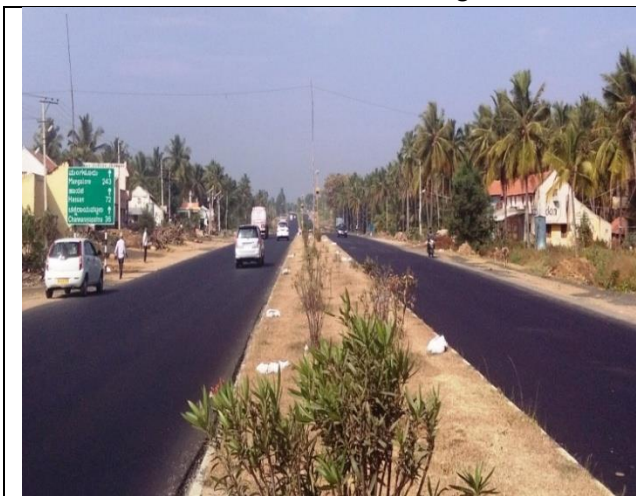
Fig. 4.1 Start Point of Project Road (At Devihalli on NH-75)
