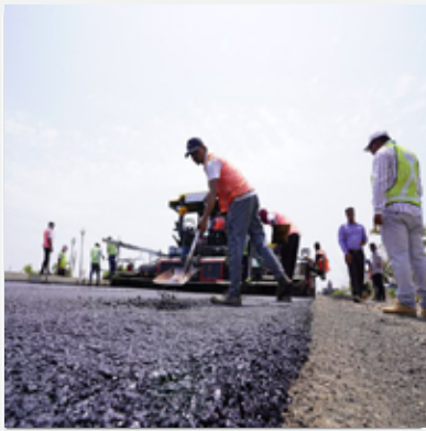
Creating World Record in National Highway Construction
