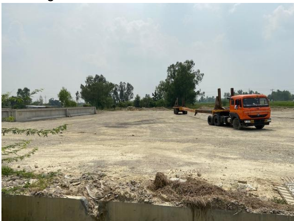
Site Internal View
