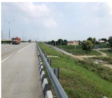
View of Access to site
