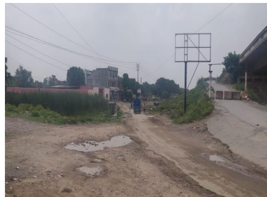
View of Site and NH -19
