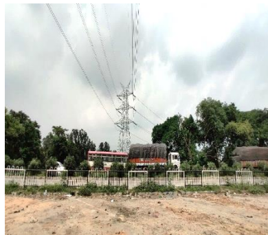
HT Line crossing from middle of the subject site
