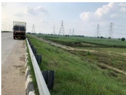
View of Access to site
