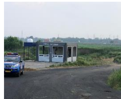
View of Access to site
