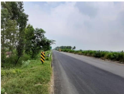
View of Access to site
