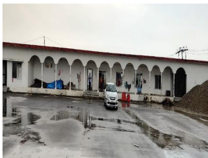
View of Built up Area
