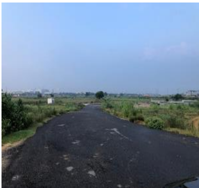
View of Access to site
