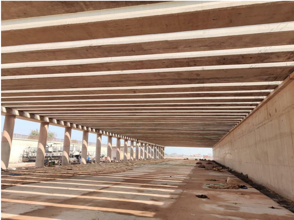
Animal Underpass constriction near Sawai Madhapur, Rajasthan
