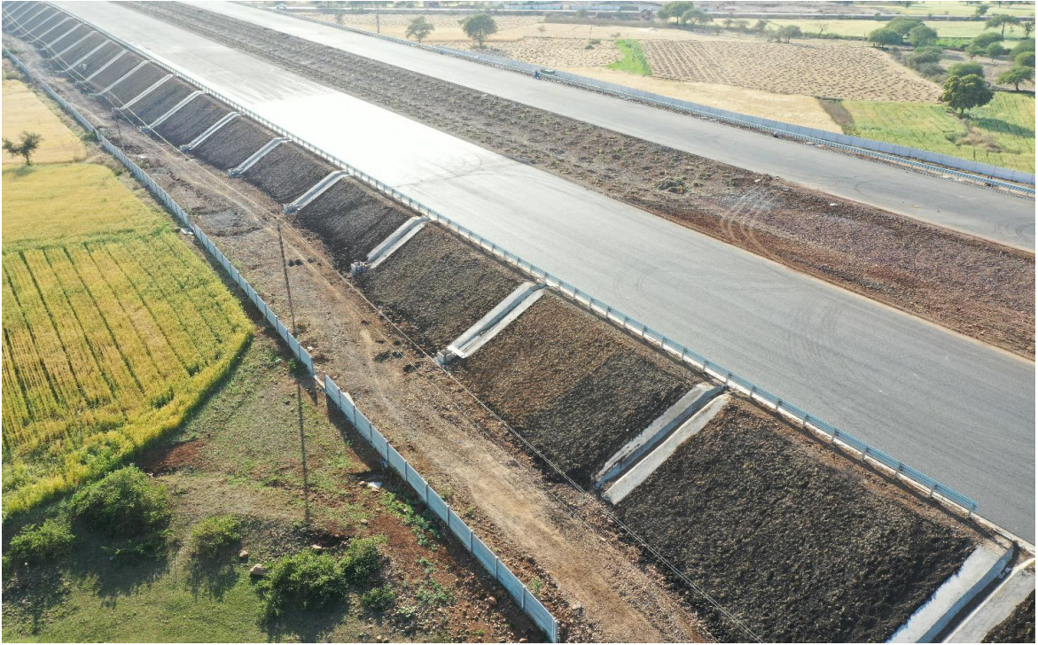
SMA completed near Ratlam, Madhya Pradesh
