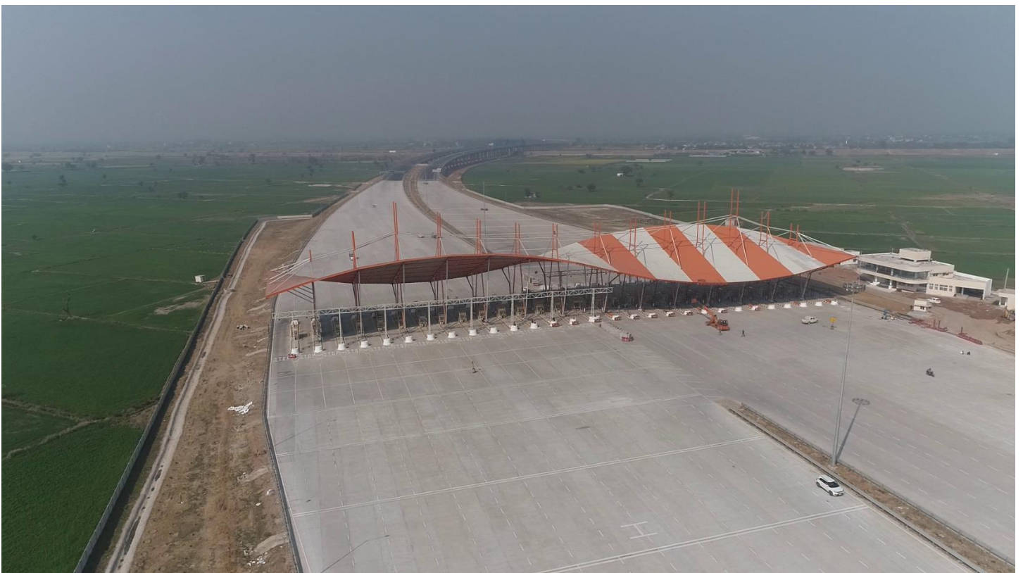
Toll plaza completed near Sohna, Haryana
