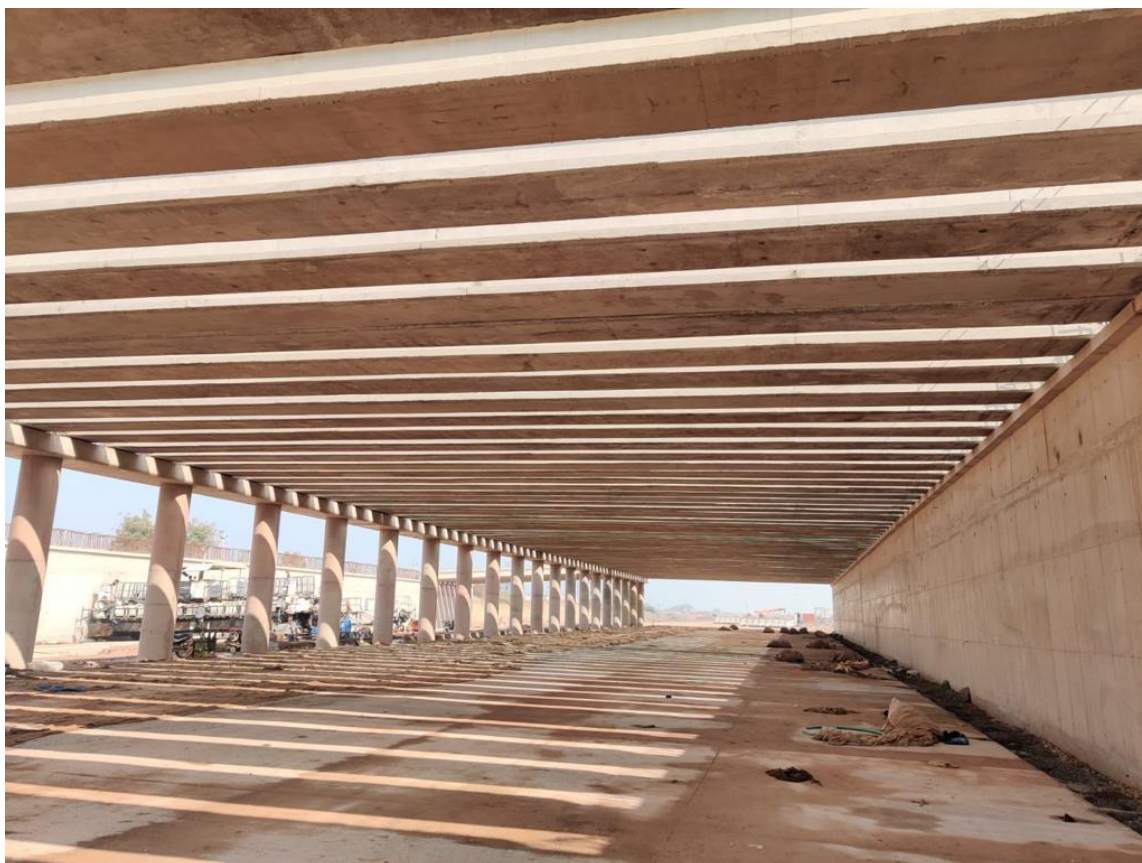
Animal Underpass constriction near Sawai Madhapur, Rajasthan
