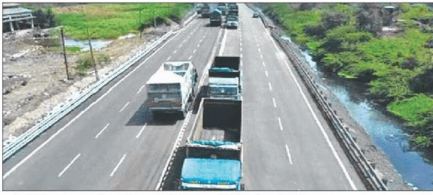
India's first six-lane bituminous steel slag road in Surat, Gujarat. CRII
