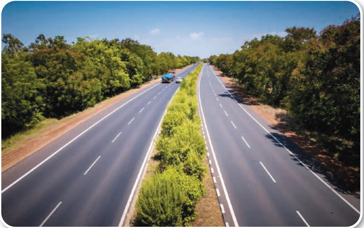
Figure 3- 4 Laning of Tada-Nellore Section of NH-16 in the State of Andhra Pradesh
