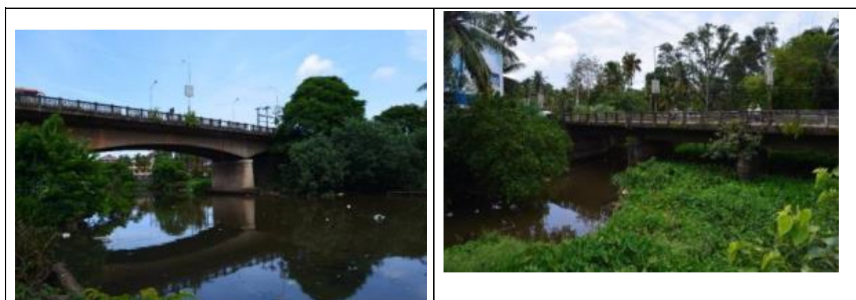
Bridge at km 458.0
