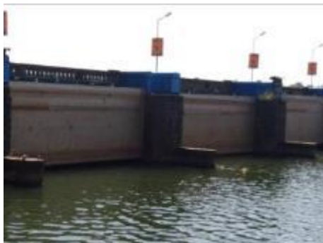
Thottapally Spillway (km 432.600)
