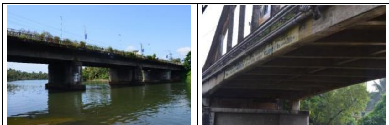
Bridge at km 474.6
