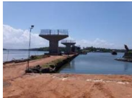
Ashtamudi Lake Bridge (km 487.200) under construction
