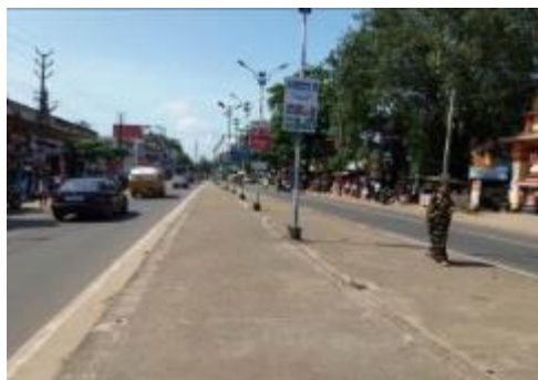
Built up/Commercial area at Karunagapally (km 470.00)
