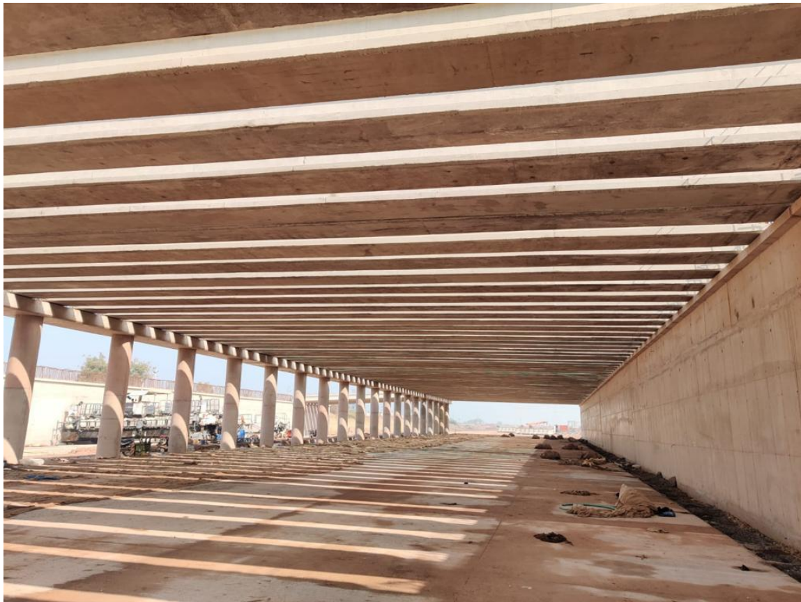
Animal Underpass construction near Sawai Madhapur, Rajasthan
