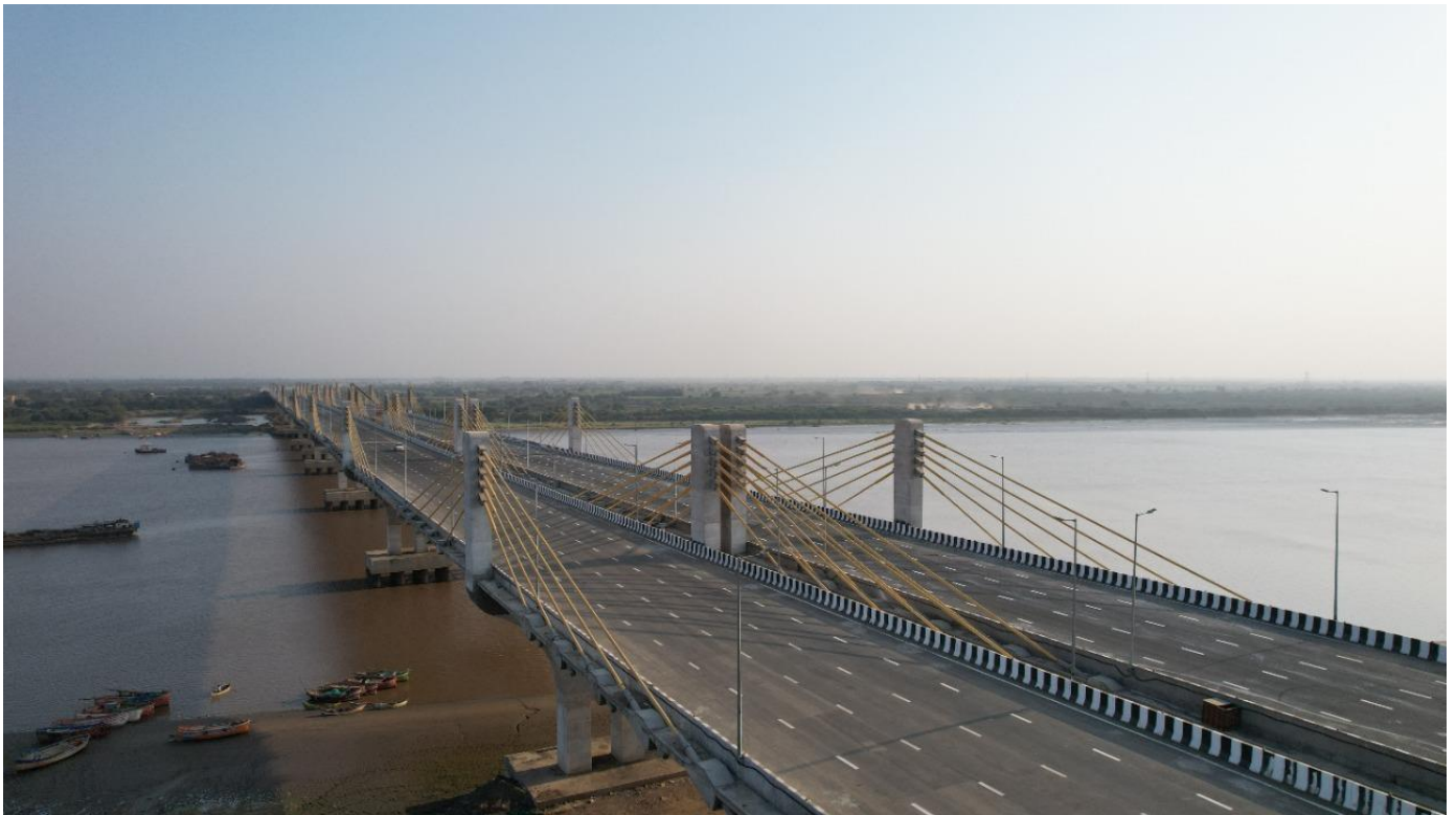
Iconic 8 lane cable stayed bridge across Narmada River near Ankeleshwar, Gujarat
