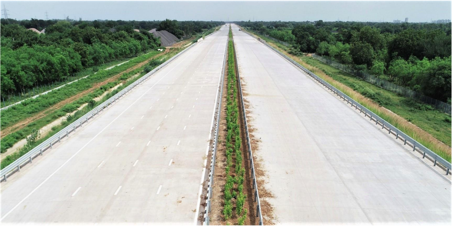
8 laning and road marking completed near Vadodara, Gujarat
