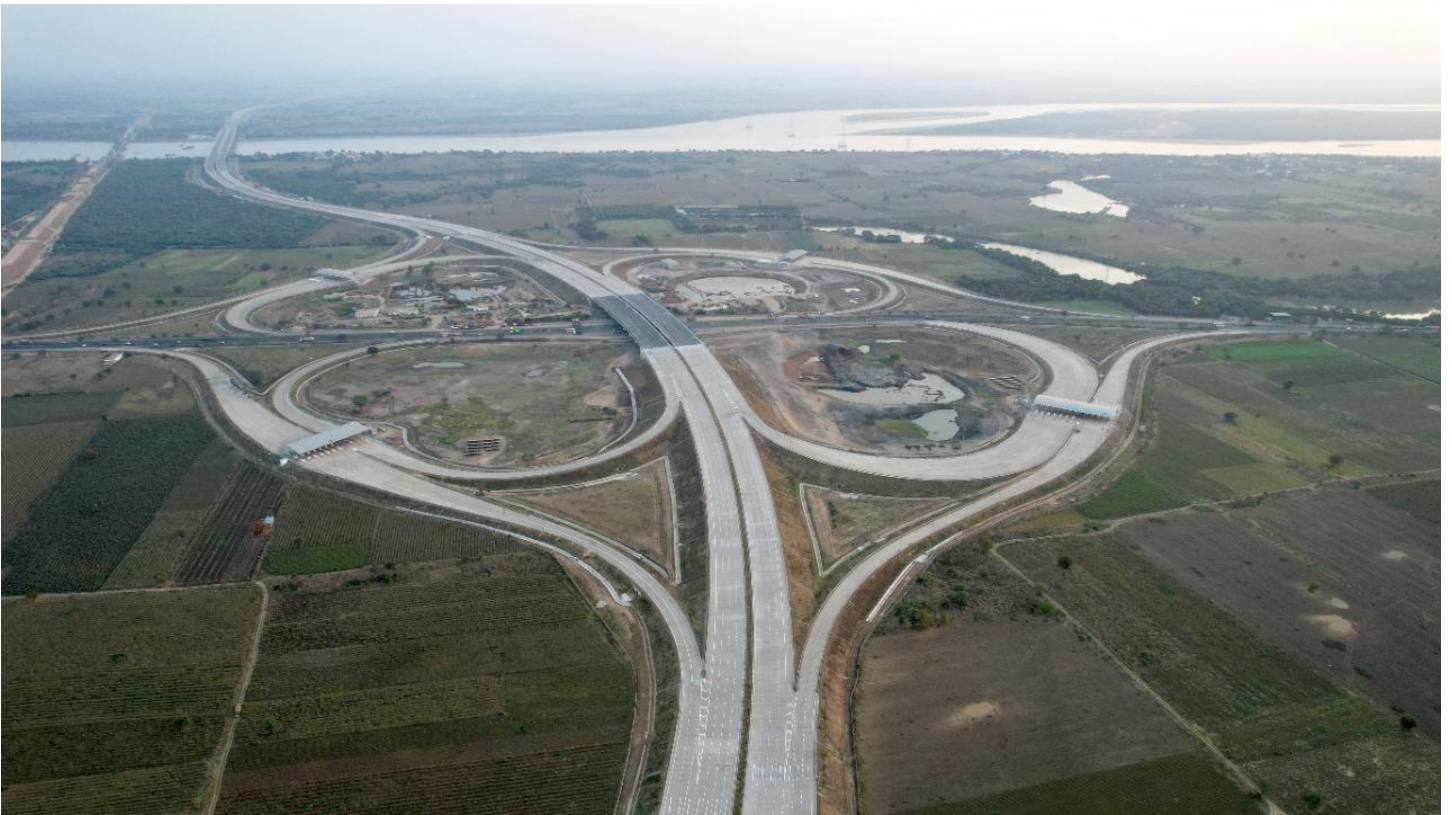
Clover Interchange near Bharuch, Gujarat
