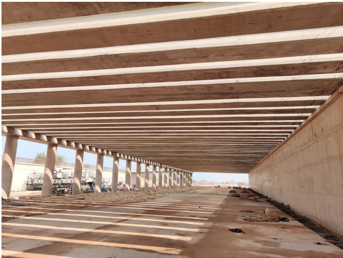
Animal Underpass construction near Sawai Madhapur, Rajasthan
