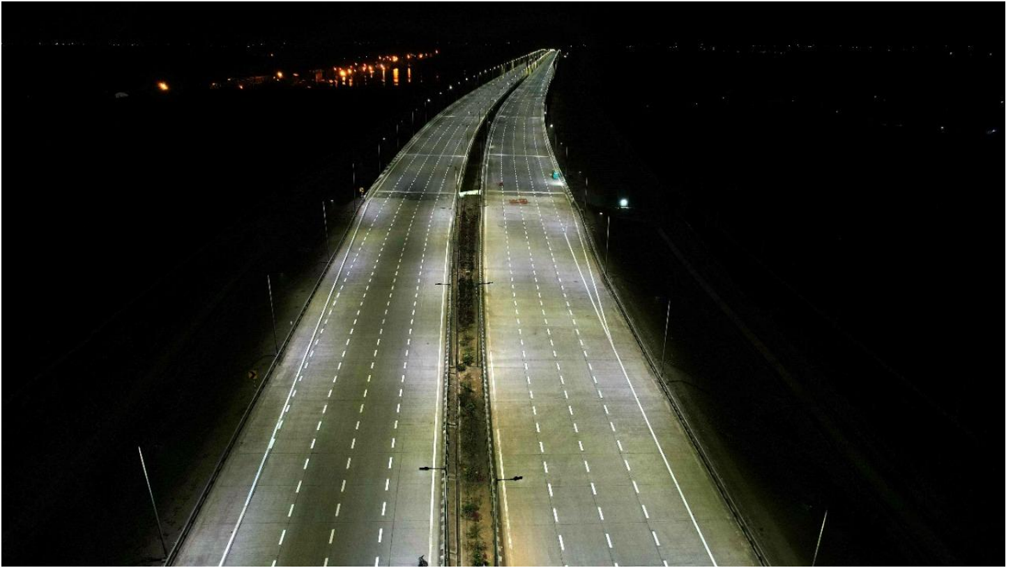
Lighting and road marking completed near Ankleshwar, Gujarat
