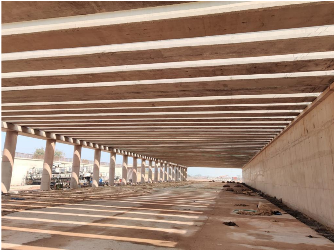
Animal Underpass construction near Sawai Madhapur, Rajasthan
