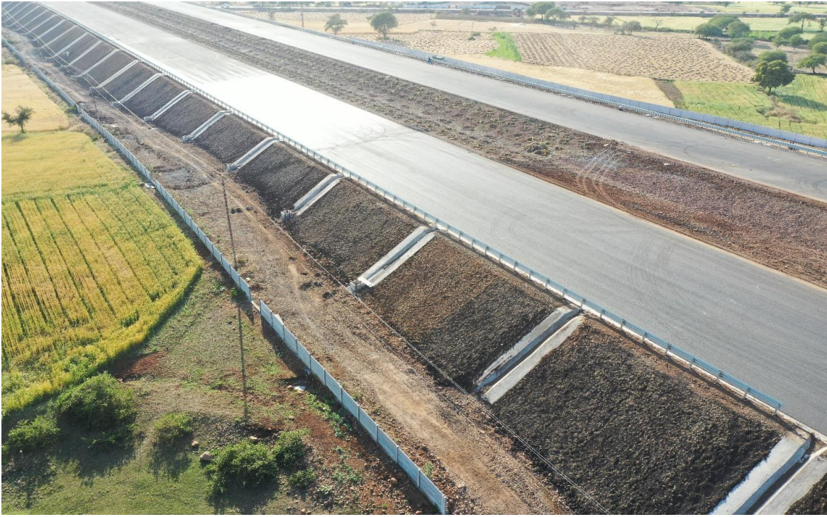
SMA completed near Ratlam, Madhya Pradesh
